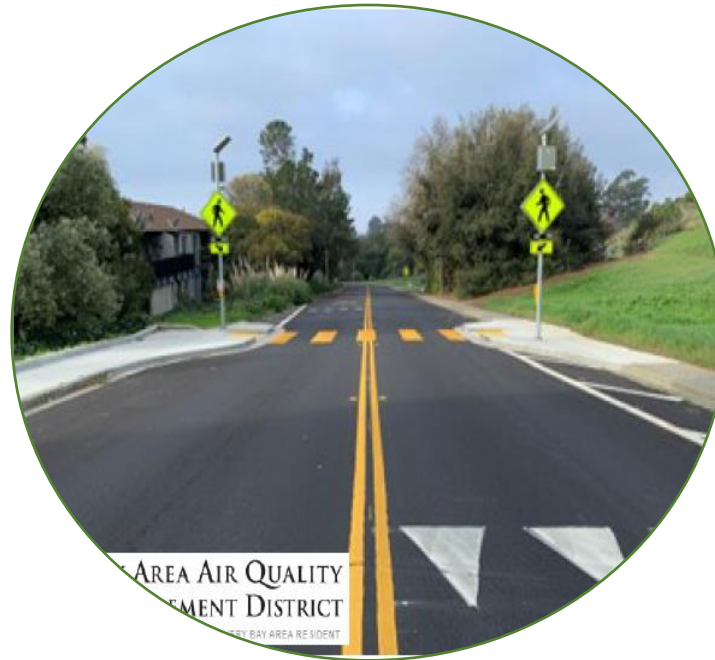
Benicia- Panorama Drive School Safety Pedestrian Crossings Improvements
