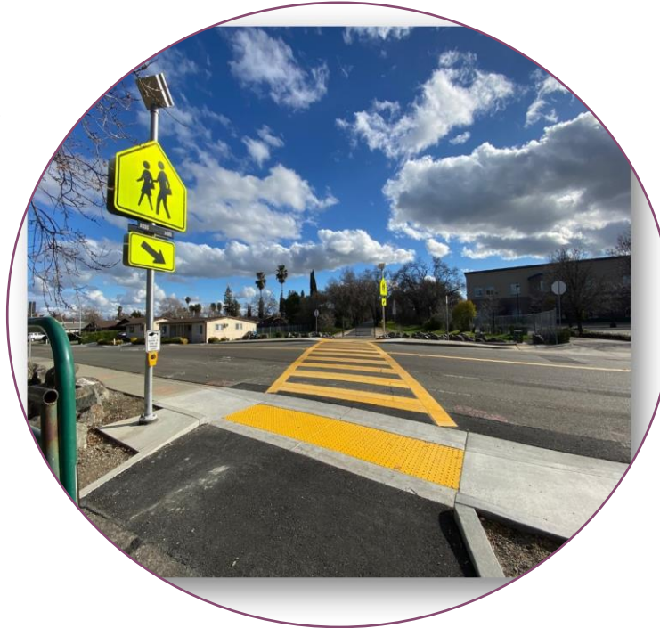
Vacaville Marshal Road Rectangular Rapid Flashing Beacons
