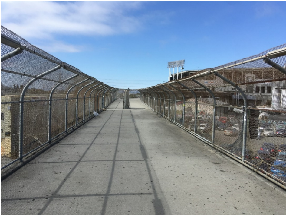
FIGURE 6 - COLISEUM CAPITOL CORRIDOR PEDESTRIAN BRIDGE (USERS' VIEW)
