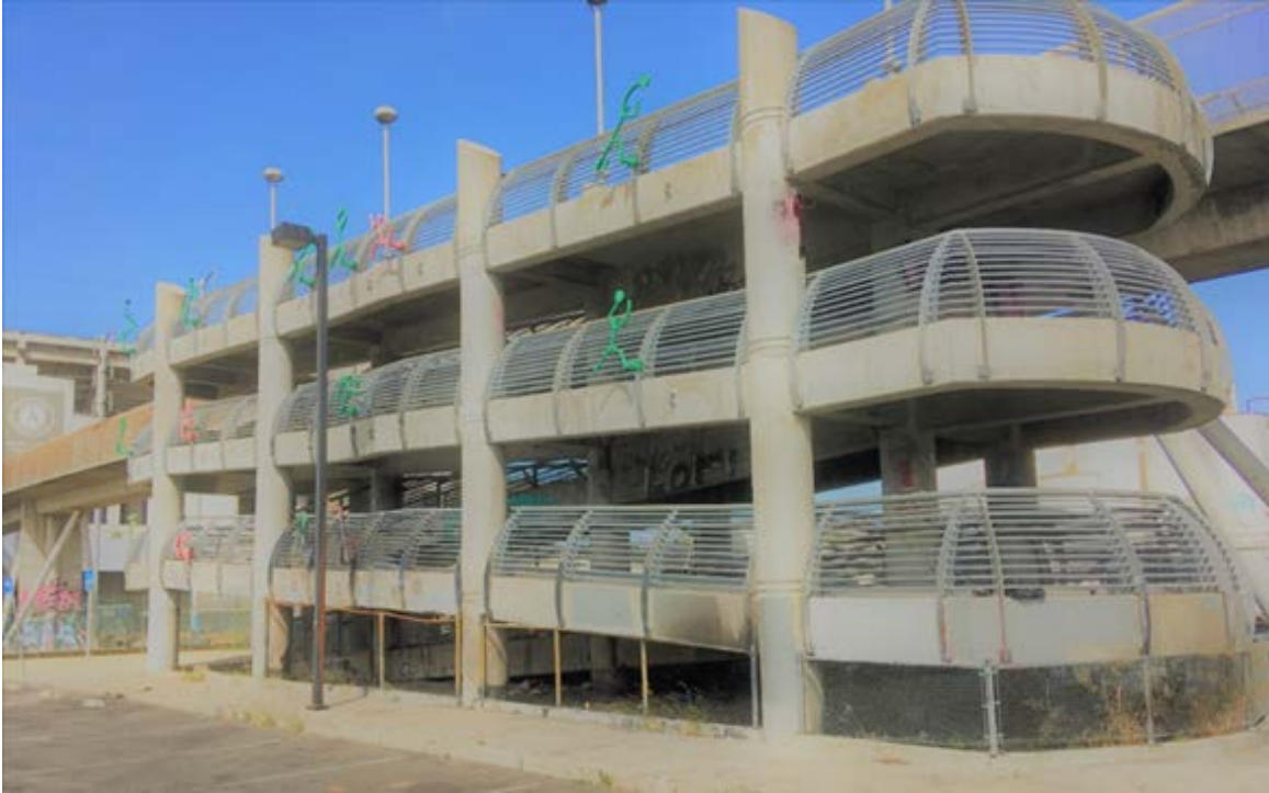
FIGURE 7 - COLISEUM CAPTORL CORRIDOR PEDESTRIAN RAMP
