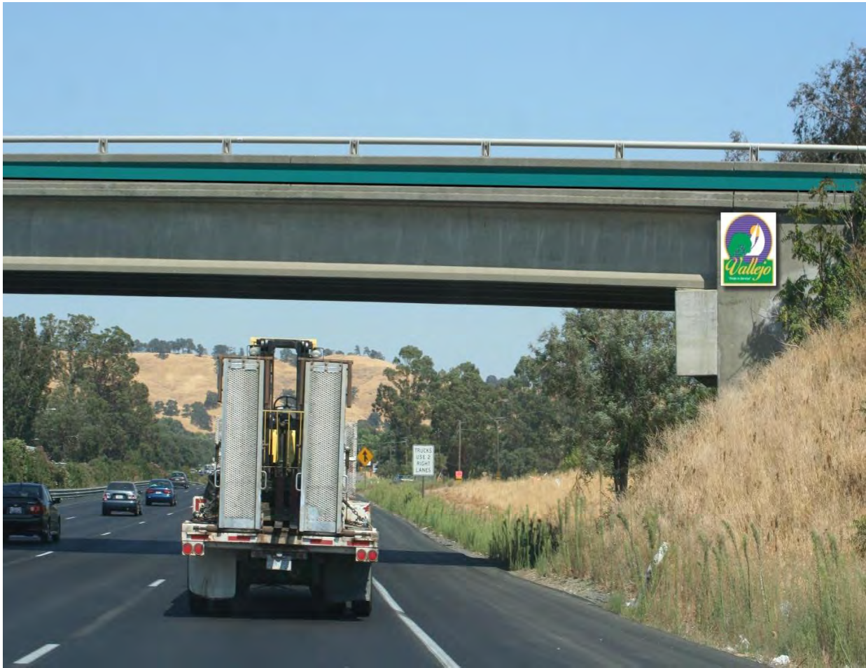
Vallejo Overpass Gateway Treatment
