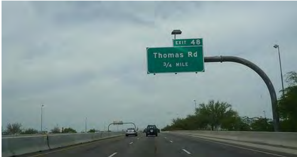
Highway Signage Support Structure Treatment
