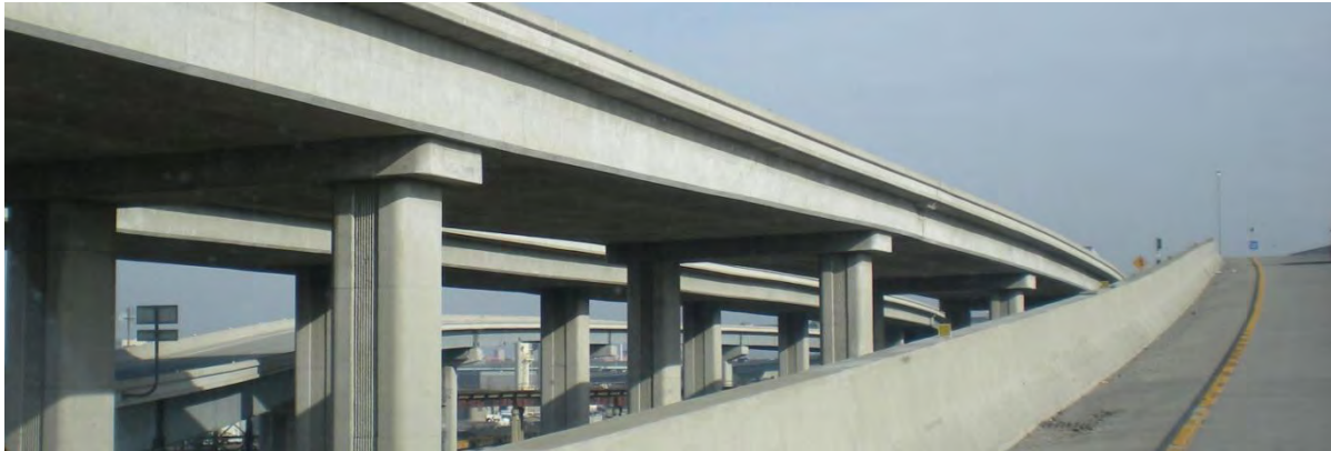
Bridge Structure Treatment
