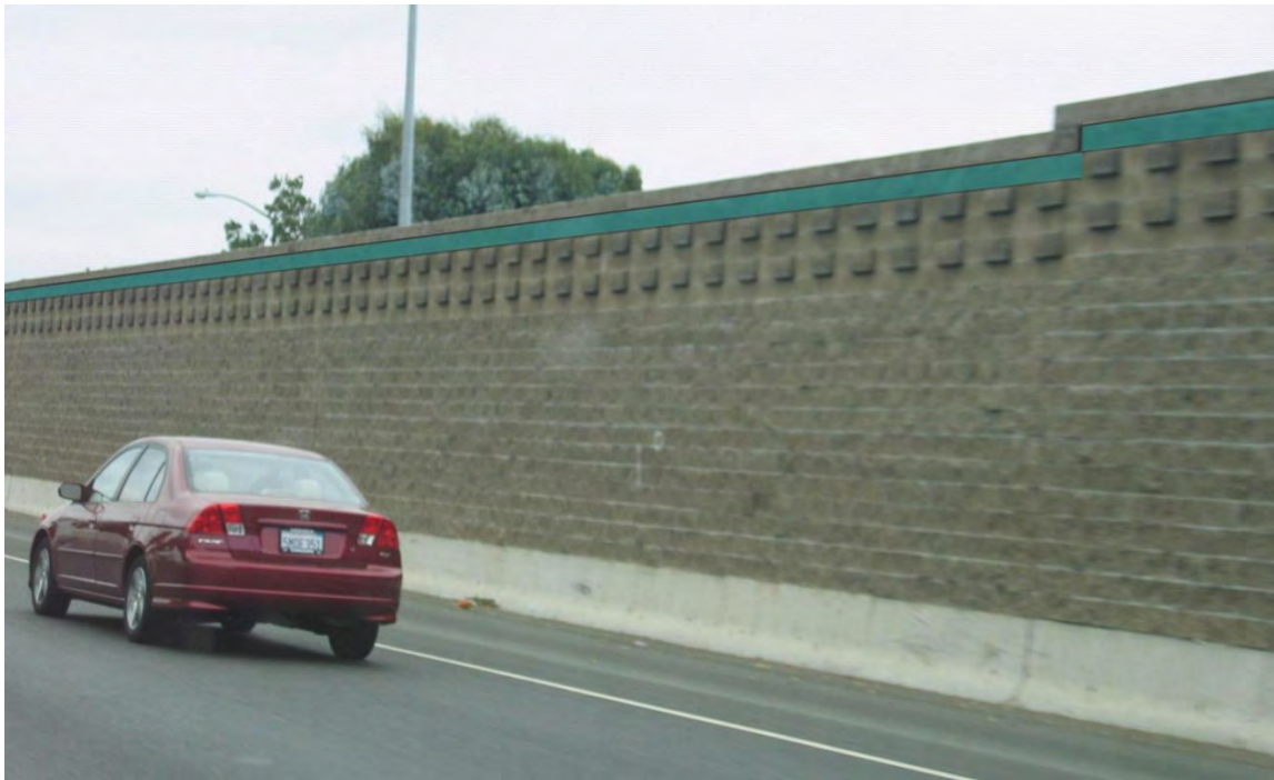
Sound Wall Treatment
