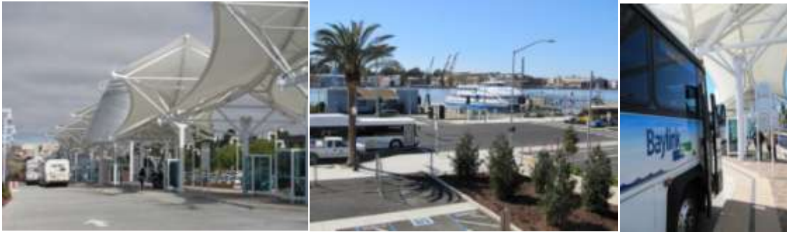
Vallejo Transit Center: The attractive new Transit Center links the downtown bus terminal to the ferry, though it can be up to a ¼ mile walk between the two. A 1,200 space free parking facility for the ferry is being constructed between the two. (Photos: Courtesy of Mike Jones)
