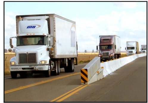
SR 12 Temporary Median Barrier
