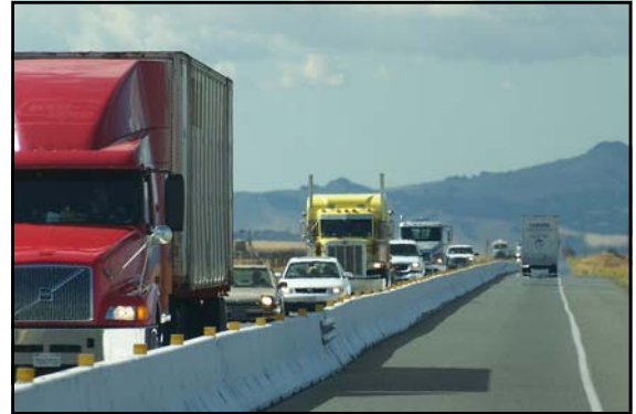
SR 12 Temporary Median Barrier
