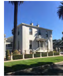
2 Jefferson Street Mansion (Lieutenant's House)(1863)
