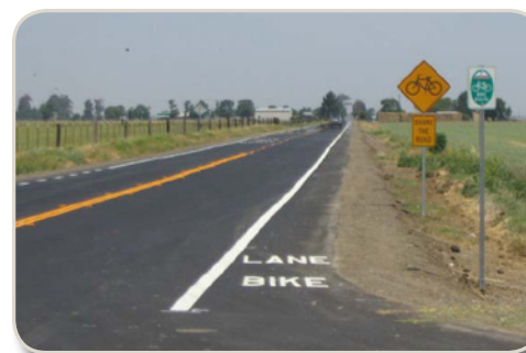
Class II Bikeway (Bike Lane) – Striped On-Street
