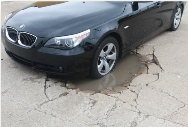
Potholes can grow into major obstacles if not treated quickly. *(Pothole not located in Vacaville)
