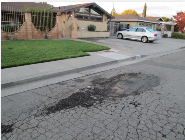
Potholes can grow into major obstacles if not treated quickly.
