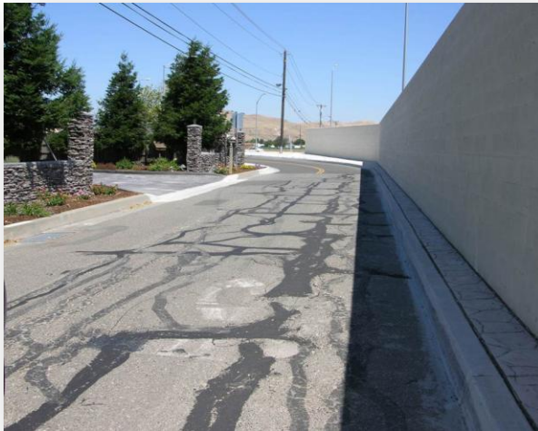
At-Risk/Poor Pavement Condition
