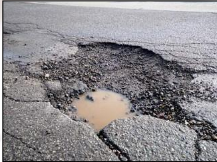
Figure 1: Pothole Example
