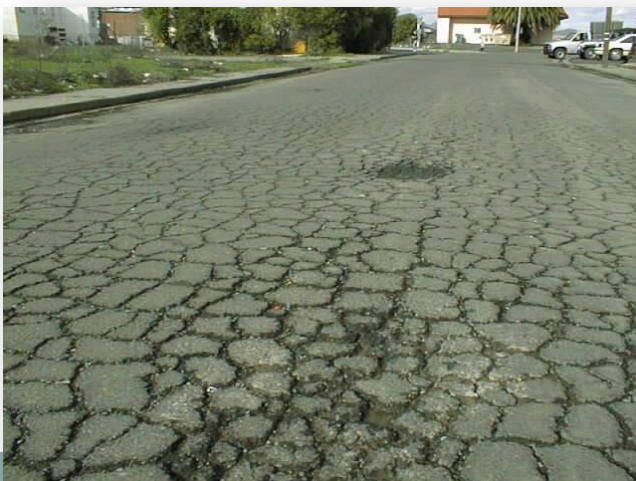
Poor/Failed Pavement Condition
