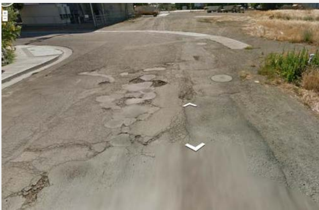
Poor/Failed Pavement Condition
