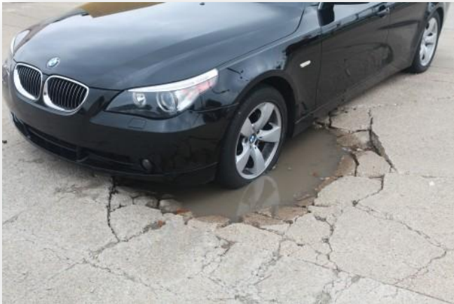
Potholes can grow into major obstacles if not treated quickly.
