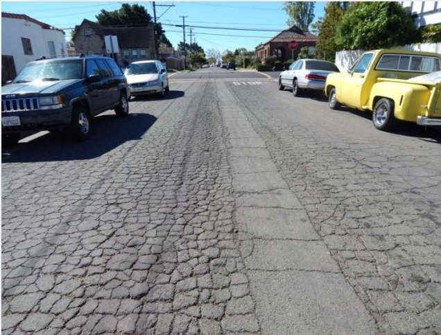
Poor/Failed Pavement Condition
