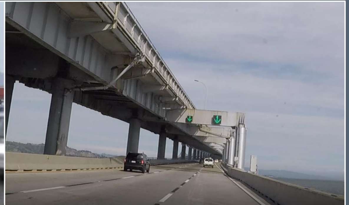
Richmond-San Rafael Bridge: Peak Period Use Shoulder Running Lanes
